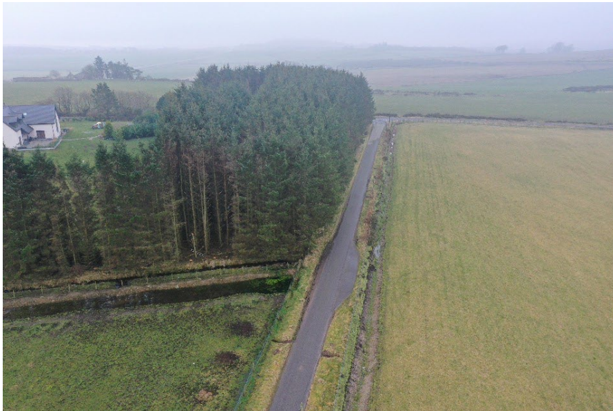
Figure 2 Aerial view of ponding at drainage outfall
